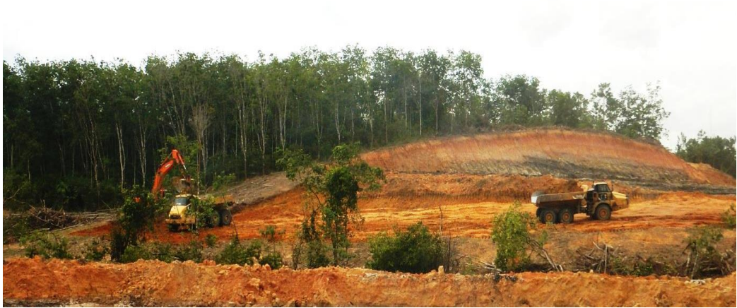
Gambar 1. Proses topsoil removal, hauling dan stockpiling
