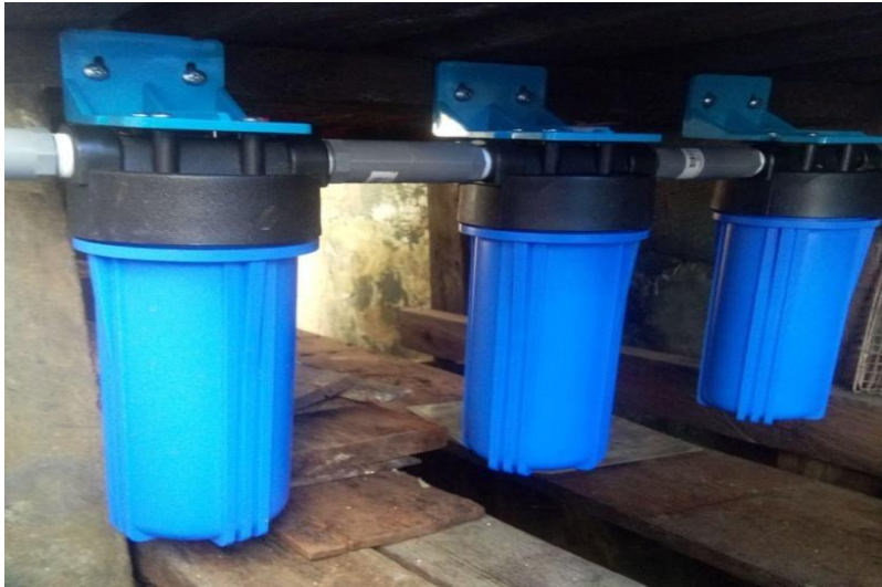
Gambar 10. Filter Air ( Cartridge filter )
